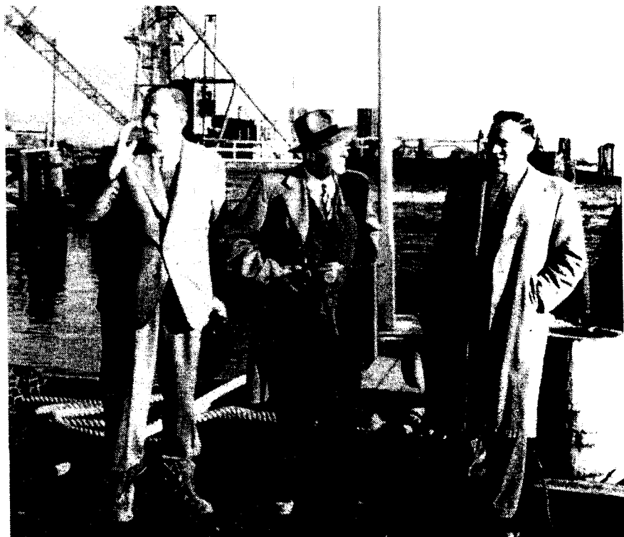
Figure 20. Karl Terzaghi (centre) inspecting construction of Deas Island Tunnel (now George Massey Tunnel).
