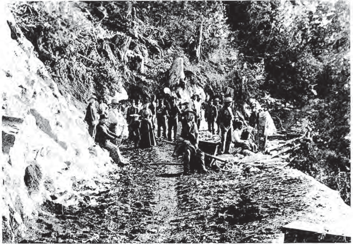
FIG. 10. The only known photograph of the Cariboo Wagon Road under construction. The exact location and date are unknown; however, it was probably taken in 1862 along the Thompson or Fraser River (B.C. Archives photo 74225).
