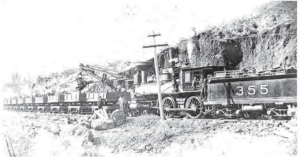
FIG. 16. An 1896 photograph of a CPR work train and steam shovel just north of Drynoch landslide (B.C. Archives photo 61335).
