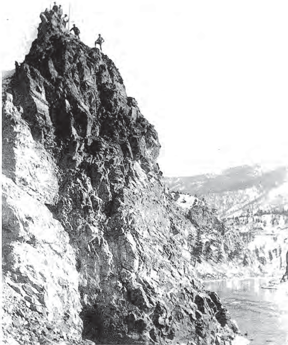
FIG. 17. A Canadian Northern Railway survey party, surveying along the rugged west bank of the Thompson River near Drynoch landslide. Photograph was taken in 1911 (B.C. Archives photo 30150).
